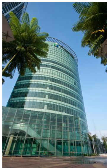
Tropicana City Office Tower, Petaling Jaya
